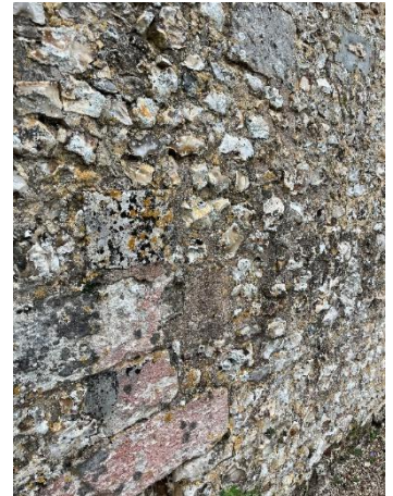
A wall at Bec Abbey
